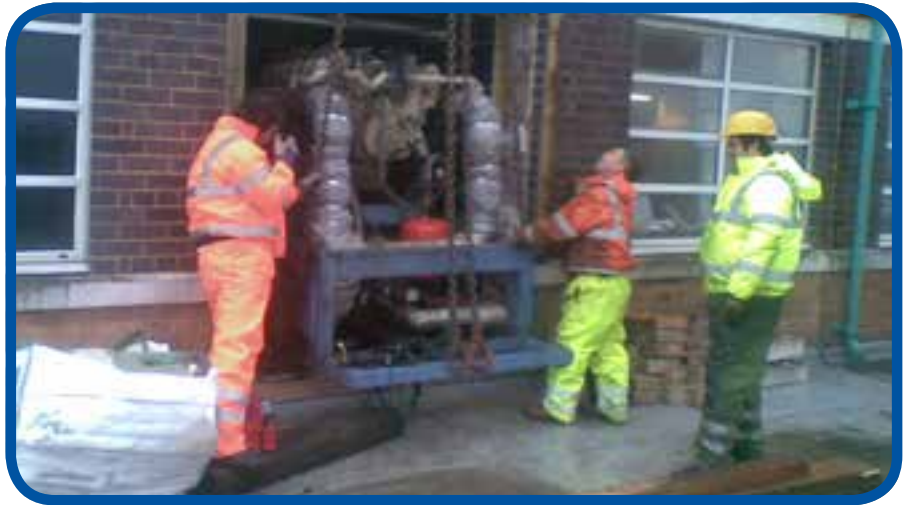
Careful installation at the Crowne Plaza Hotel
