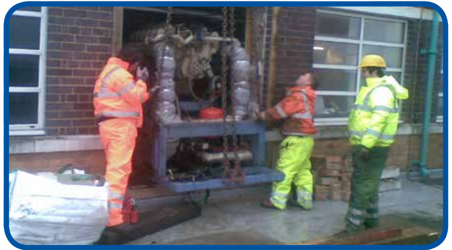
Careful installation at the Crowne Plaza Hotel
